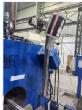
IR Pyrometer installed near extrusion press exit
